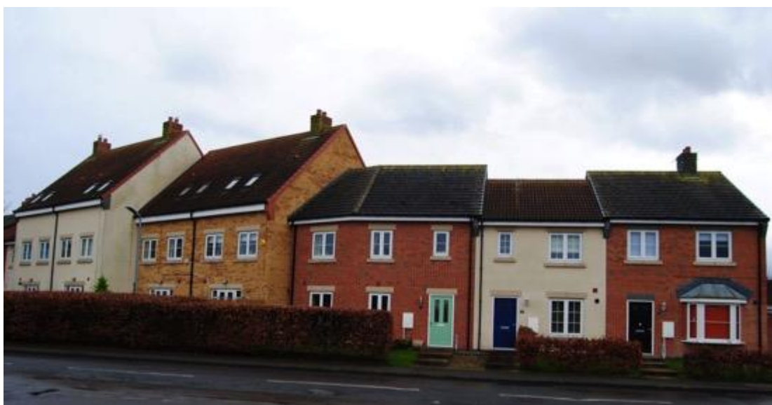
Good design of terraced housing, addressing site with distinct design and positive boundary treatment.
